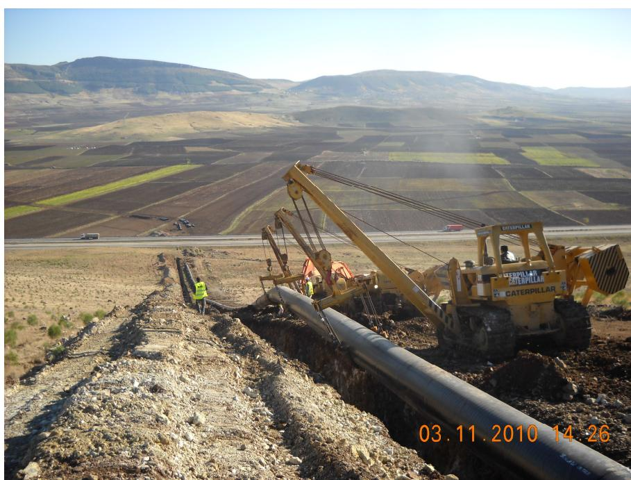
**Hatay Natural Gas Pipe Line Construction 16", 36" 157.767m**
